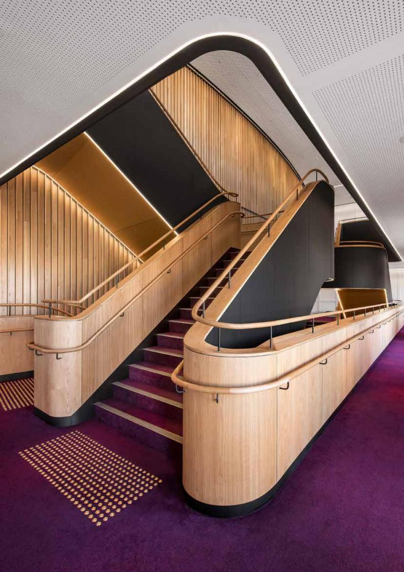
design team to successfully create the challenging, complex curved theatre forms. The veneer panels were crown cut, allowing Reuther to deal with the complex curves in the joinery geometry, giving a consistent finish as the panels curved.
